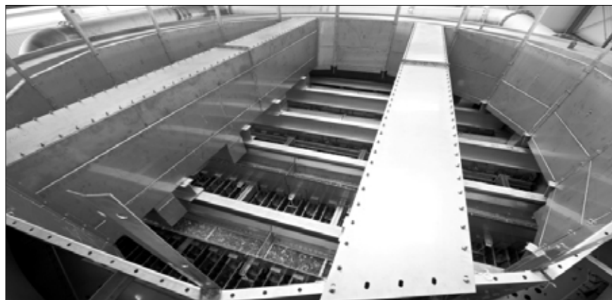
Figure 5 Large scale flash gallery and distributor at Raschig's test facility in Germany
