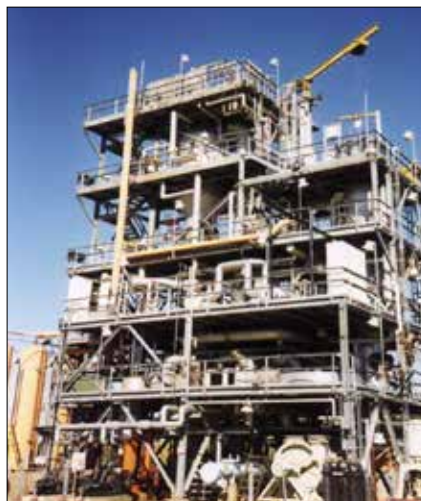
Figure 1 FRI facility for testing random packings, structured packings and trays under industrial scale conditions; left: low pressure column D = 1200 mm; right: high pressure column D = 1200 mm
